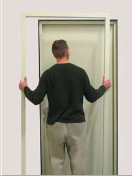
3. Frame trim piece is attached to unit and secured through the silencer holes – no exposed fasteners
